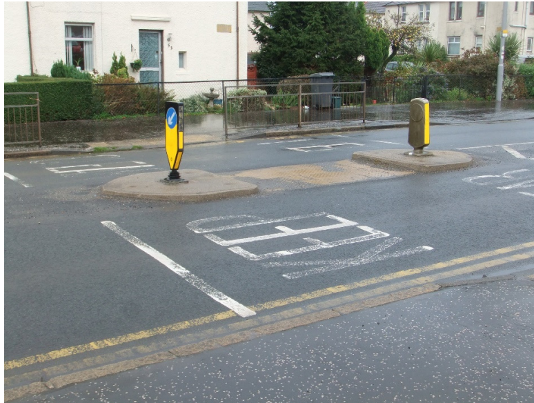
Worn markings at crossing point
