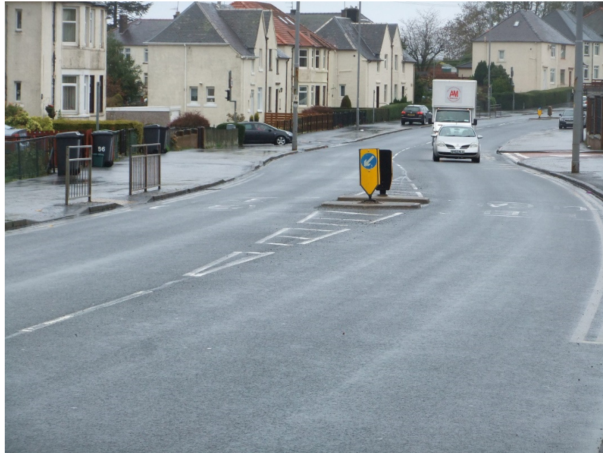
Existing keep left bollards at traffic islands
